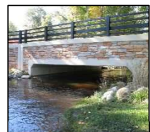
Figure 4: Three-sided box bridge
