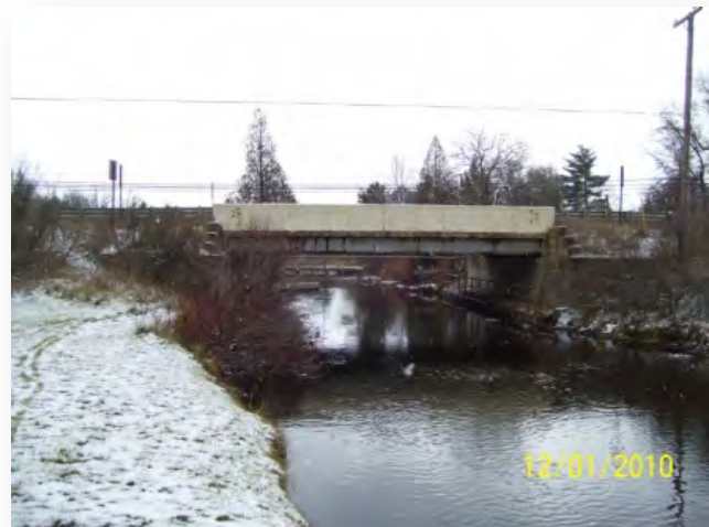
Figure 9 - North Down River Road over East Branch Au Sable River Bridge
